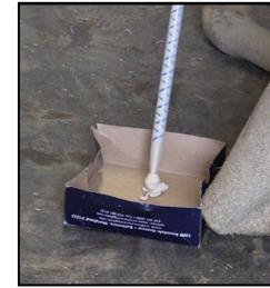
**Step 12:** Attach the mixing tube to the glue dispenser, then dispense a small amount of glue through the mixing tube to ensure the glue is mixing at the correct ratio before filling the blister.
